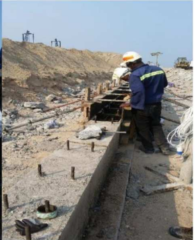
GANTRY CRANE RAIL FOUNDATION
